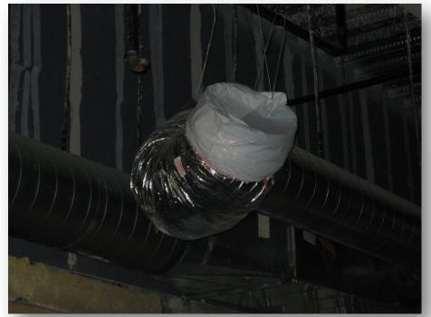
Ductwork covered to prevent dust and pest entry until system closed
