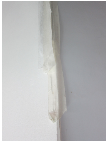
Poor taping practice
