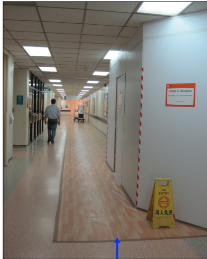
Additional layer of vinyl flooring
