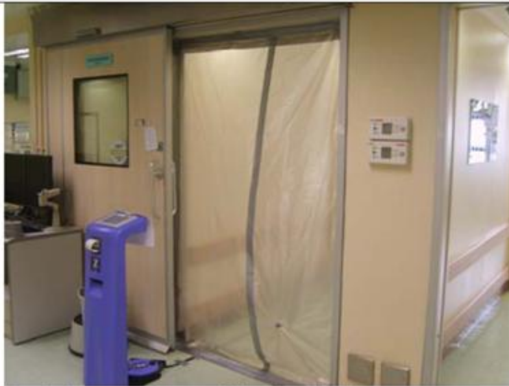
Seal the entrance with plastic sheet
