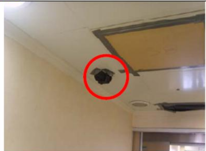
Seal the smoke detector near the entrance
