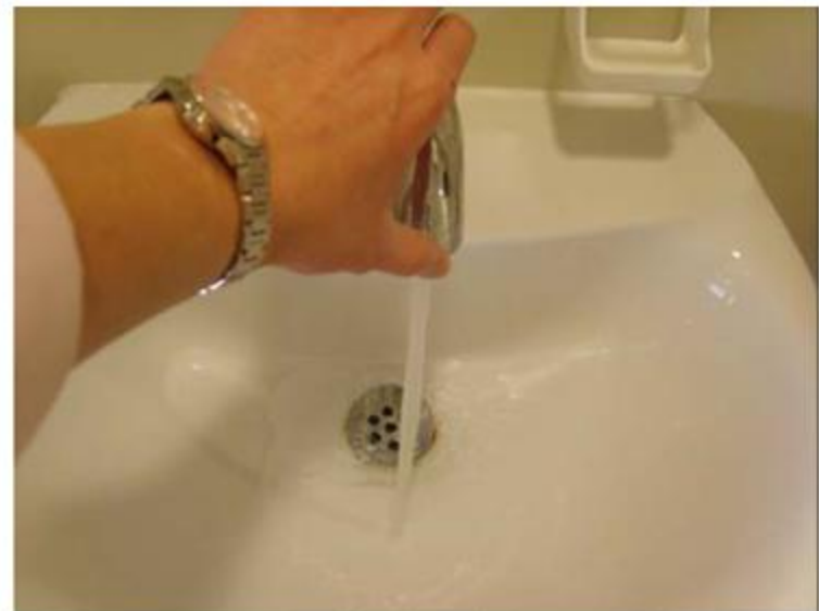
add water to the drain of the wash basin
