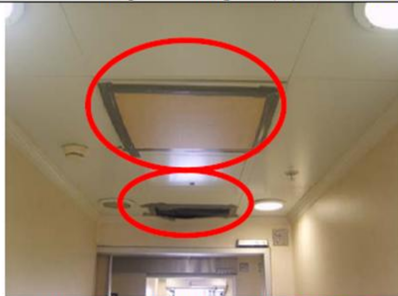
Seal the inlet and outlet near the entrance
