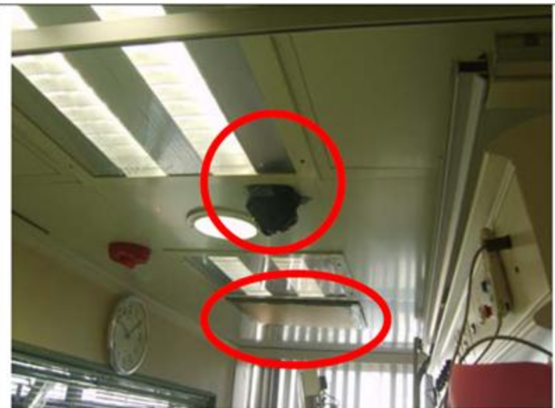
Seal the outlet & smoke detector in the room
