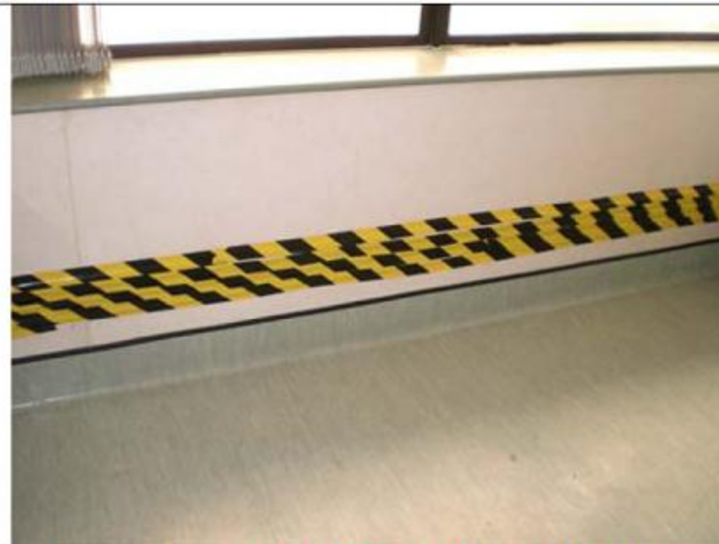
seal all exhaust grills just above the floor
