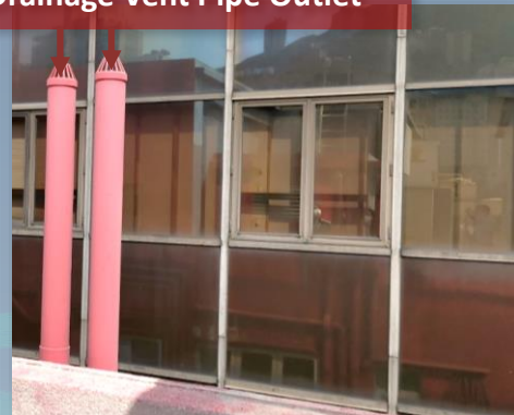
Drainage Vent Pipe Outlet
