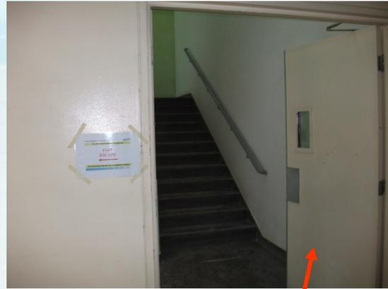
Construction site door did not close & no plywood or plastic to seal area
