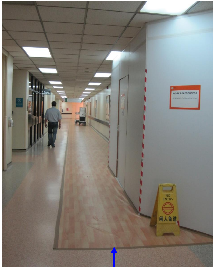
Additional layer of vinyl flooring
