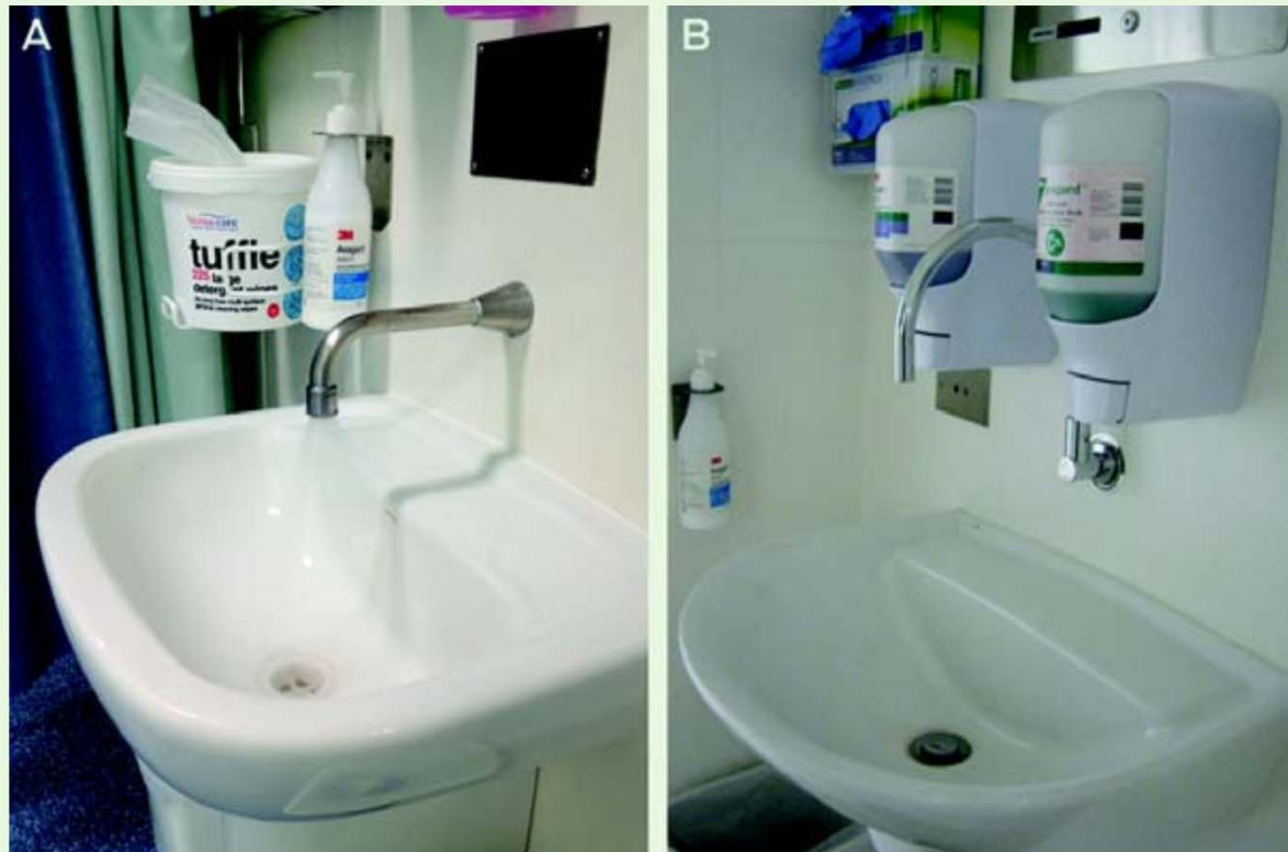
A: Existing sink, showing water spray directly over drain. B: Compliant sink design, showing larger basin and less forceful water flow directed away from drain, to prevent splash back and contamination with drain contents.
